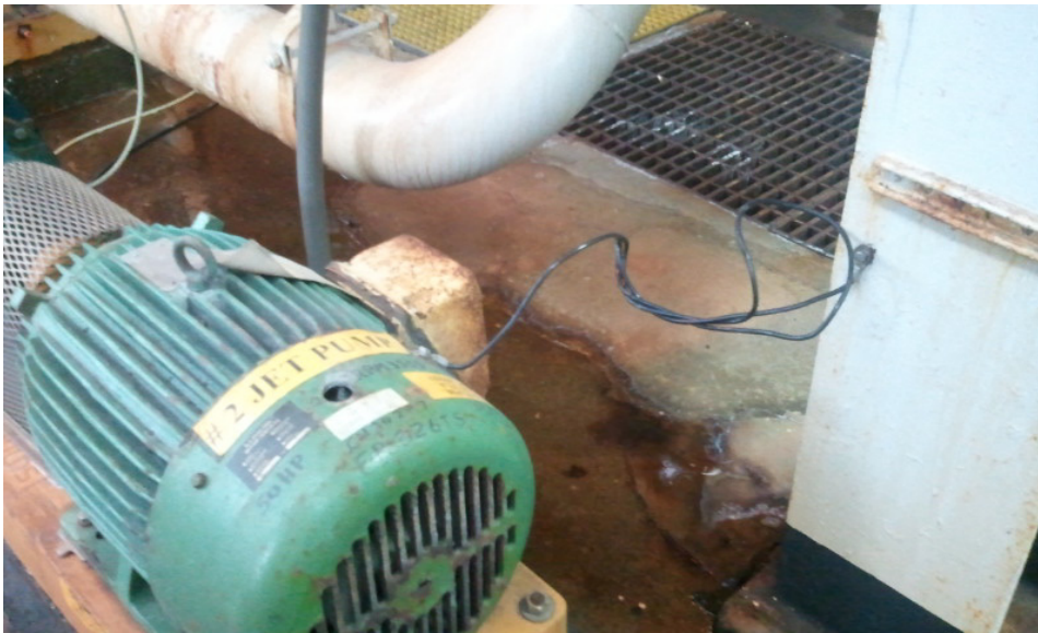
Figure 1: Motor using auxiliary ground.
